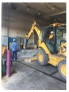
The move from JCVT to the Annex continues. In the last week of June contractors arrived to tear out concrete pads on the Annex floor to make room for tractor parking. Removal was successful. Concrete was poured on 7/1/19
