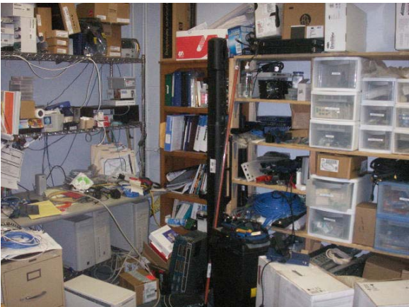
06-8 The storage and overall housekeeping in the information technology room should be reviewed. The height of the storage may make it unstable and pose a hazard while trying to retrieve the upper most items. Limiting the height of the storage
