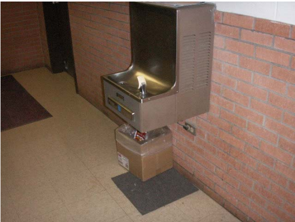
06-4 All water fountains located on tile floors should have a mat placed in front of them. This should catch any water that escapes the catch basin and reduce the potential for slipping type accidents.
