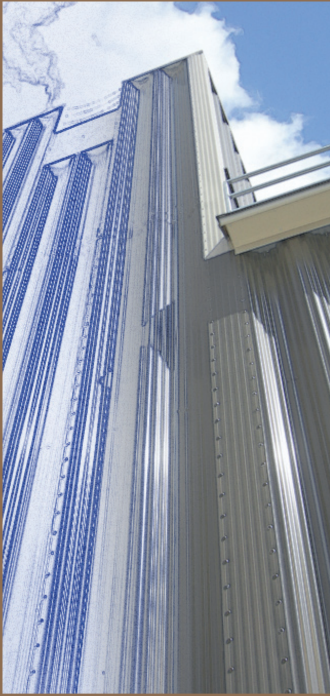
Fire tower section of the Southwest Kansas Fire Training Center, opened in 2008.
